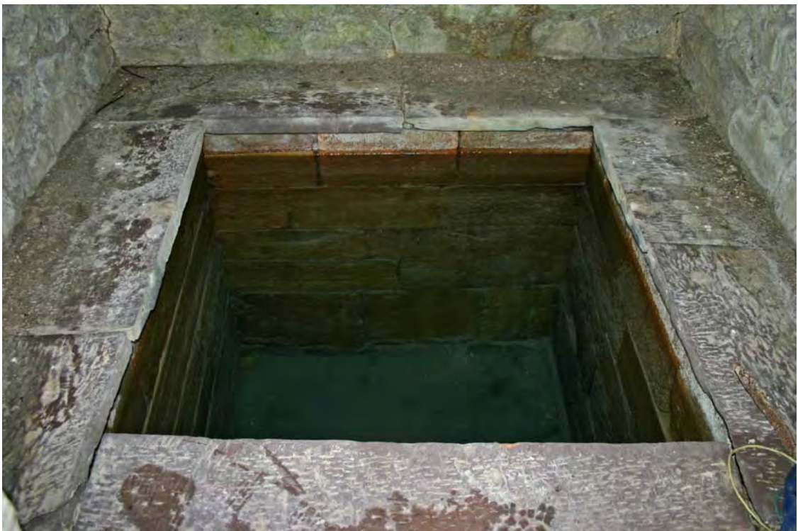
Fig 6.4 Stone lined Cistern inside the conduit head building.
